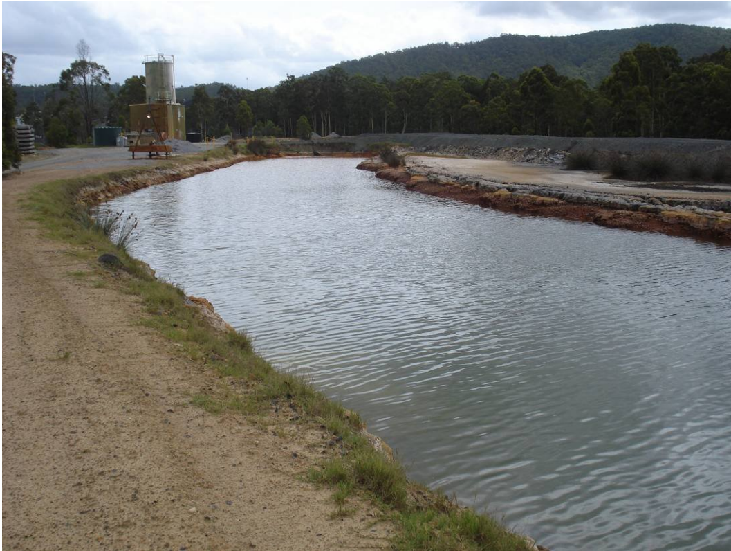
Plate 31 – Dam (in water circuit) used to settle out fines after the water from the underground has been treated through the lime plant. Note the lime plant (upper left)
