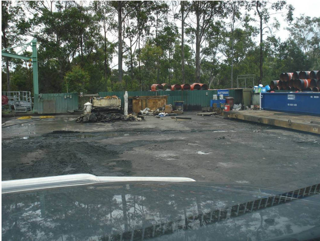
Plate 21 – General Waste and Wash down areas. Waste was placed on the pad and sorted (centre) into the bins (right)
