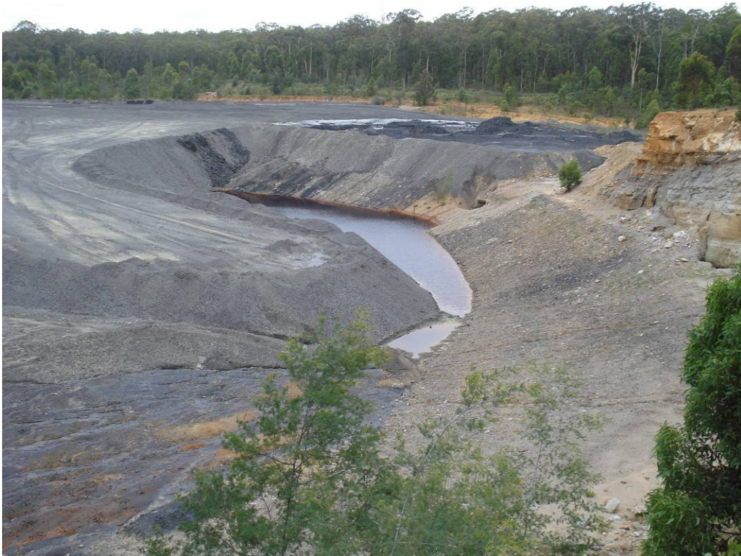
Plate 26 – Rejects emplacement area. Water accumulating in this area drains back into the underground mine eventually returning to the longwall. The pH was apparently <2.
