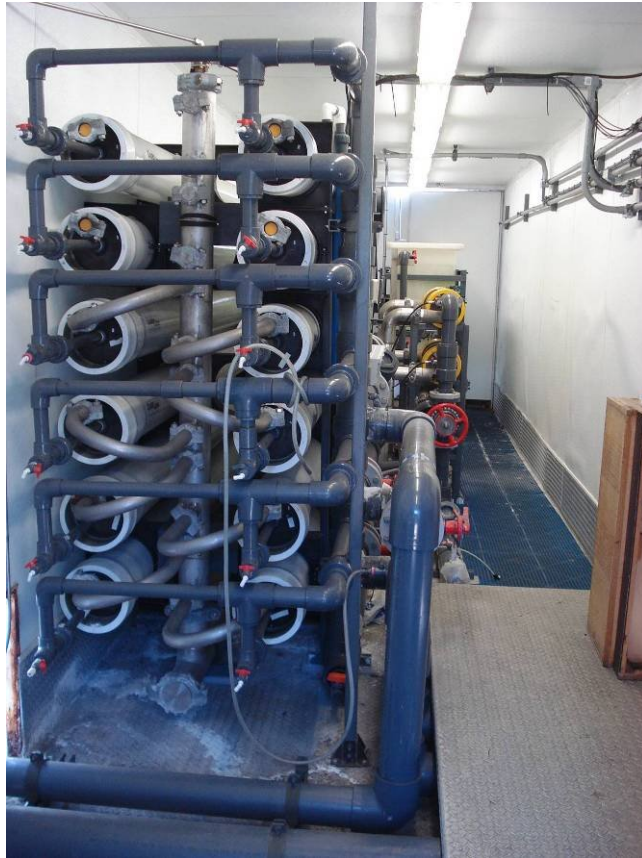
Plate 13 – The Reverse Osmosis Plant used to treat water from the Underground
