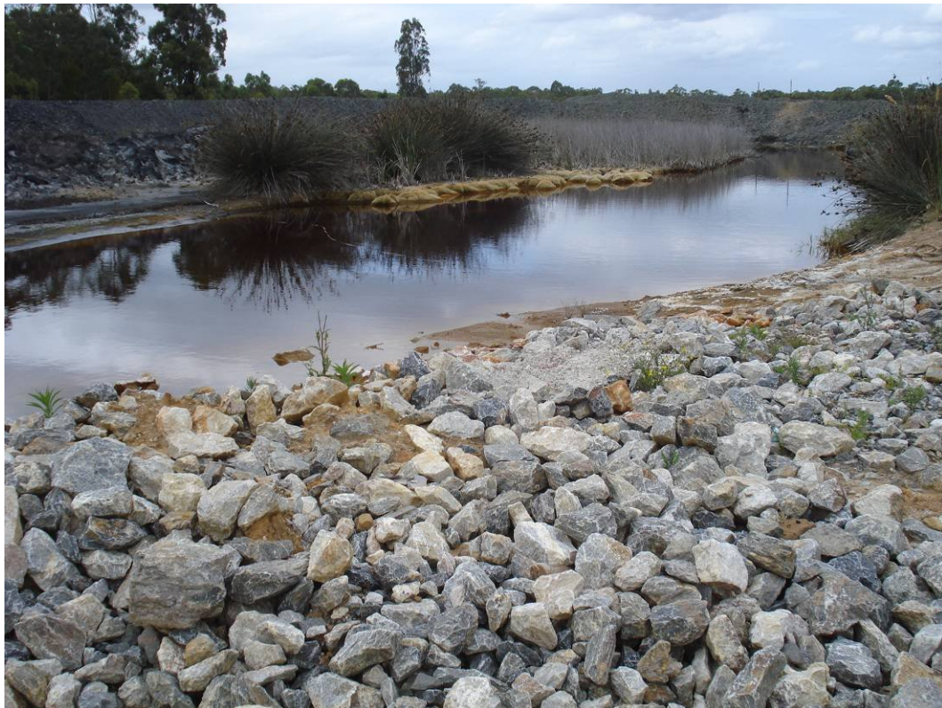
Plate 34 – Water quality after it has been passed through the lime plant and completed a circuit of the settlement dam. Water is then pumped to a dam before being treated in the RO Plant and discharged from the site.
