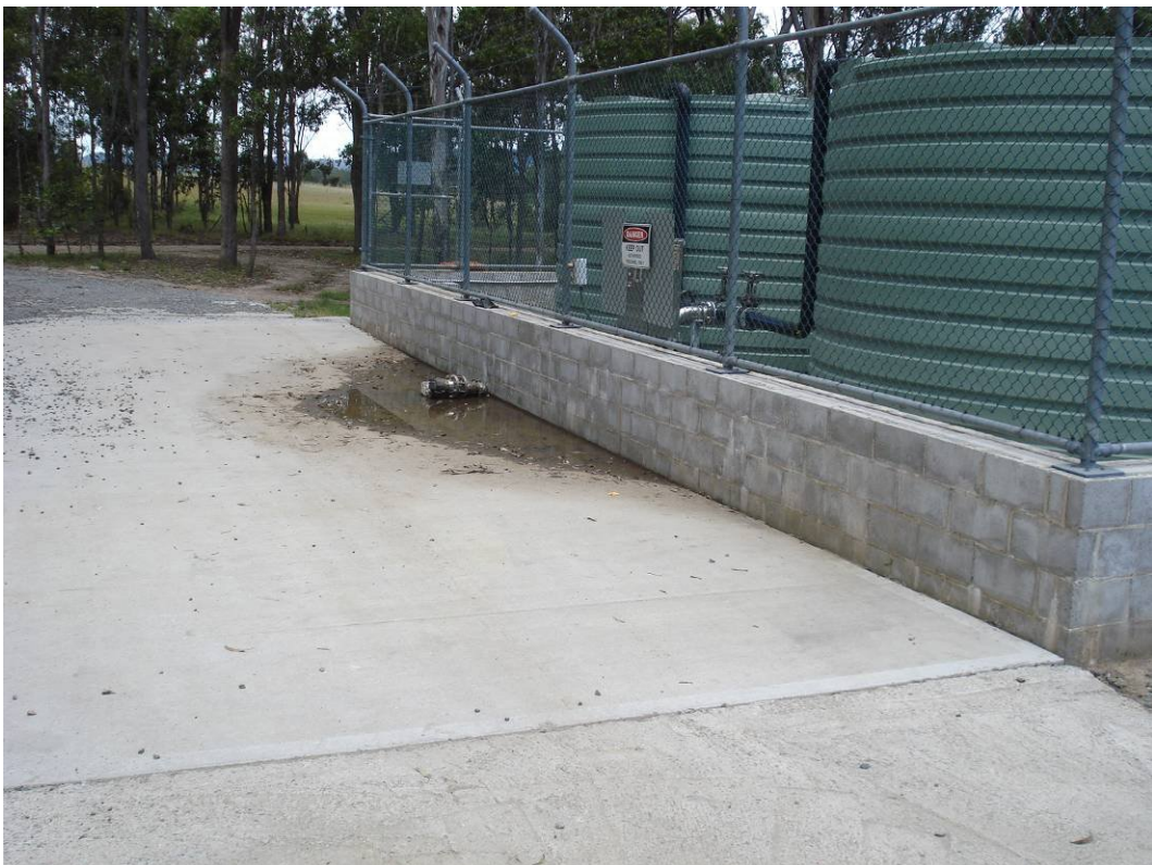
Plate 8 – Solcenic Tanks filling point. Tanks have bunding, although water collecting on this pad is drained back into the bunded area.
