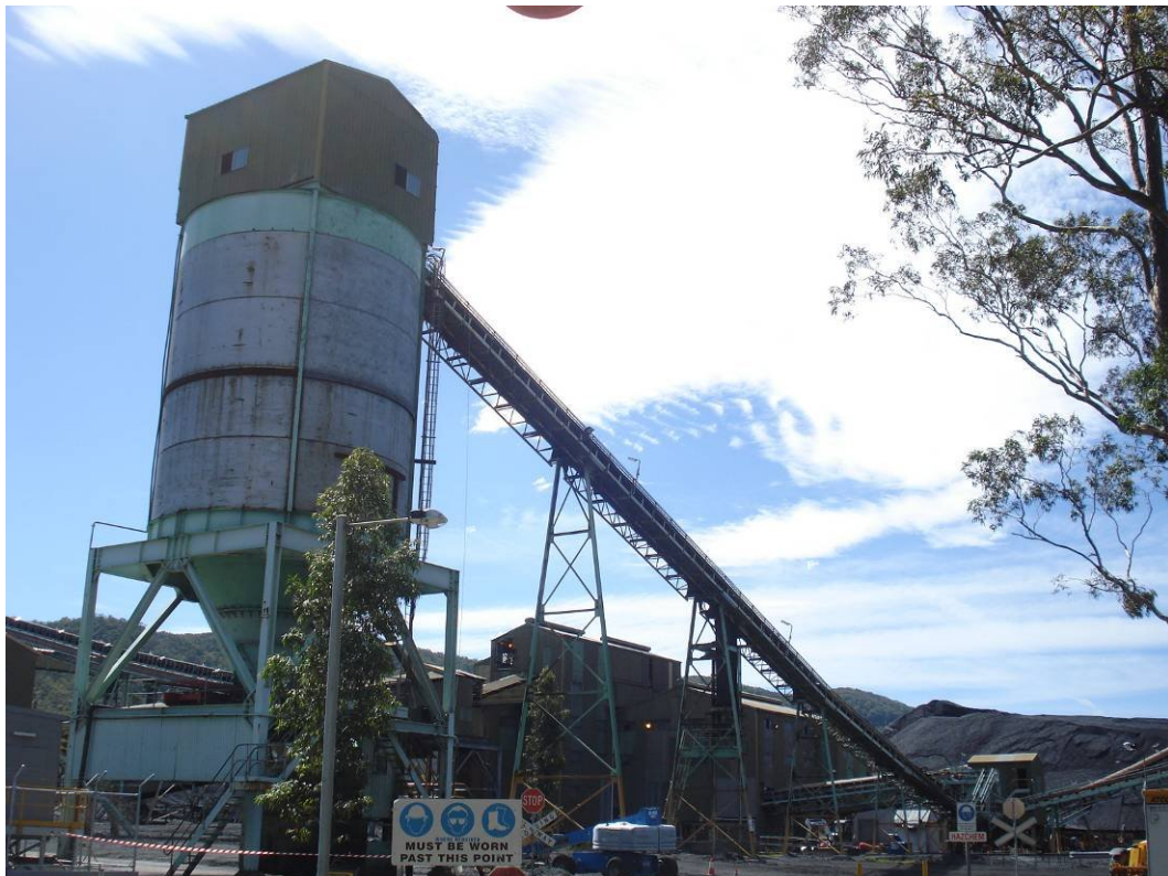
Plate 14 – Product Bins and conveyors at the Coal Preparation Plant
