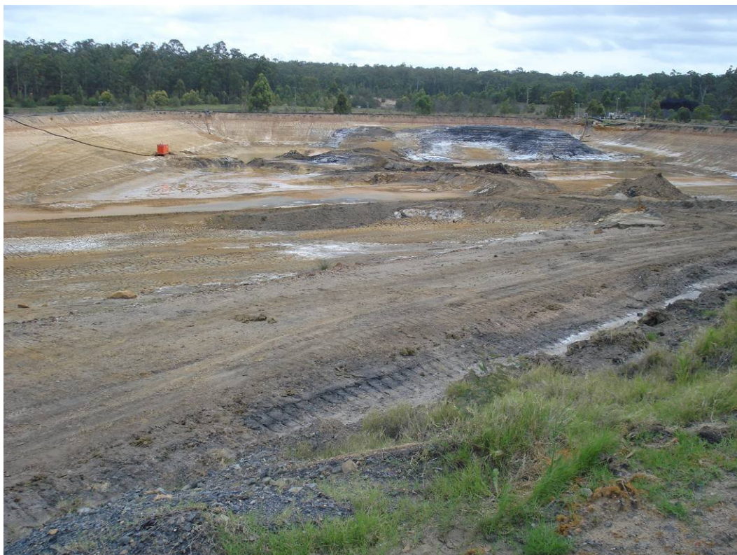
Plate 30 – An old tailings dam that is being cleaned out. At the time of the audit it was Austar's intention to utilise the dam for additional site water storage.
