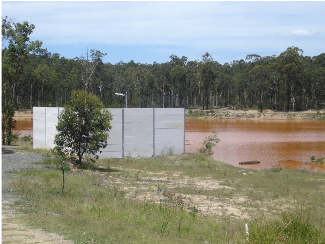
Plate 6 – Kallingo Dam with noise mitigation bunding around the pump. Note the orange colour in the water is a results of iron oxide
