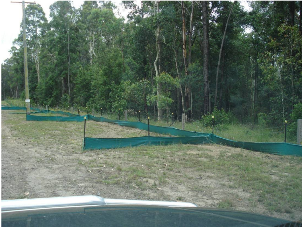
Plate 17 – Erosion and sediment control fencing adjacent to the main office
