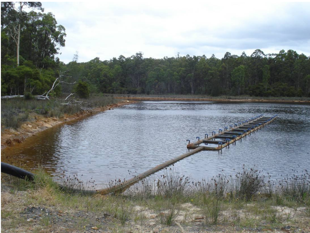
Plate 24 – Austar dam below the main offices and pit top area. Water from this dam is sent back via overland pipe to the Coal Preparation Plant
