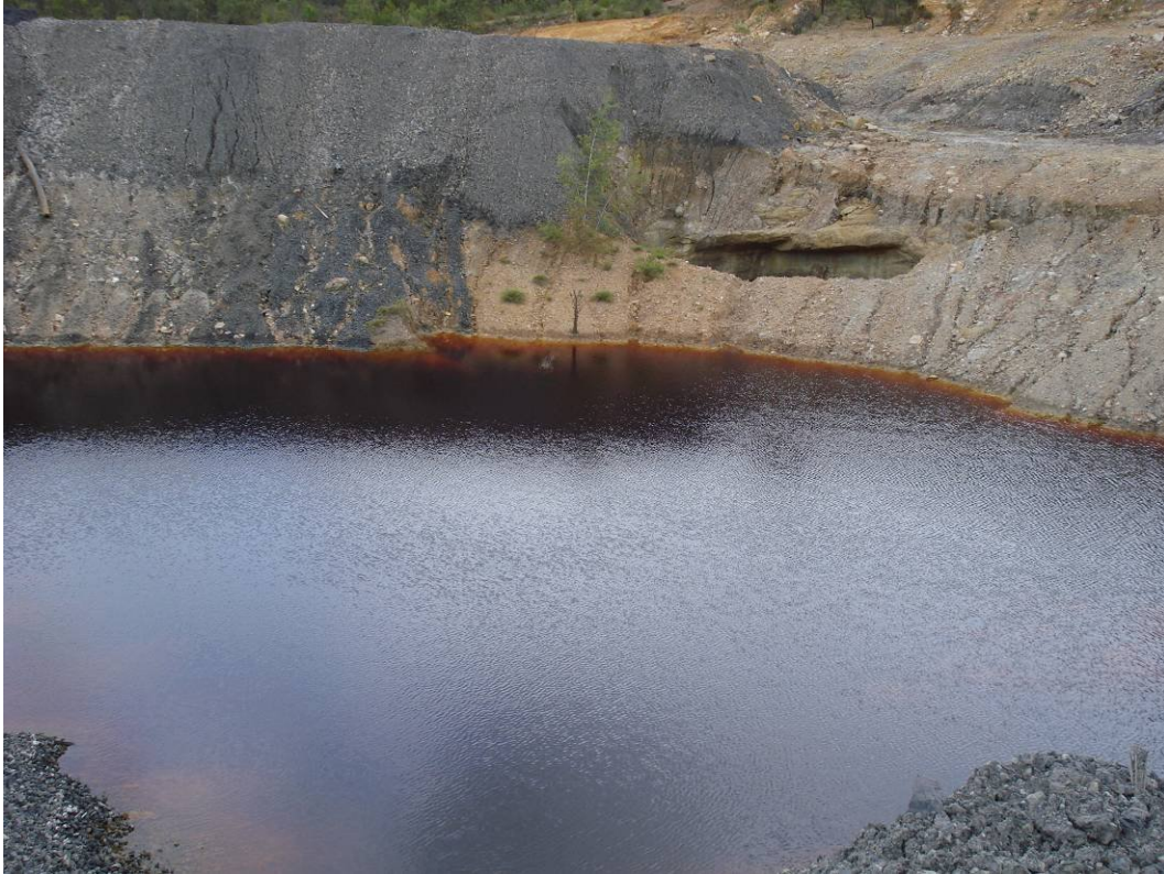
Plate 27 – Run off and leachate accumulating below the reject emplacement. Note the old shallow underground workings have collapsed and day lighted – water draining back into the workings
