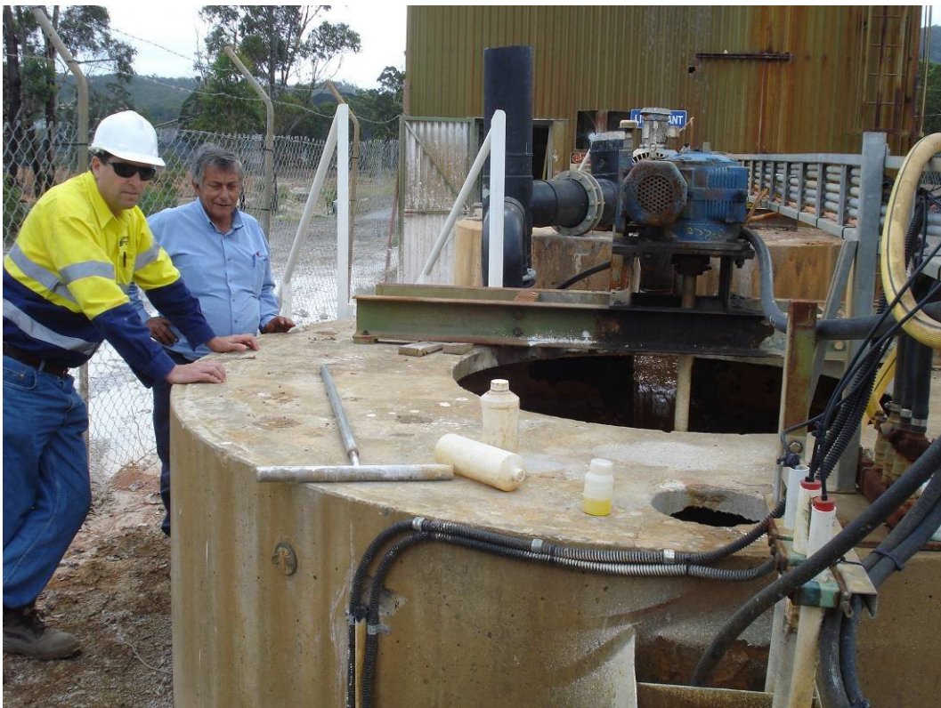
Plate 32 – Water being mixed with a flocc prior to being treated in the lime plant
