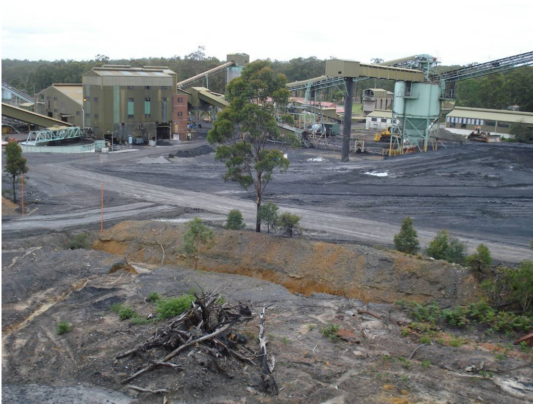
Plate 35 – General view from the rejects noise bund back towards the coal plant
