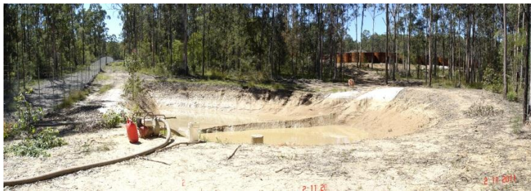
Plate 4.6C: Sediment basin east of the watercourse collecting runoff from the materials storage and handling area.
