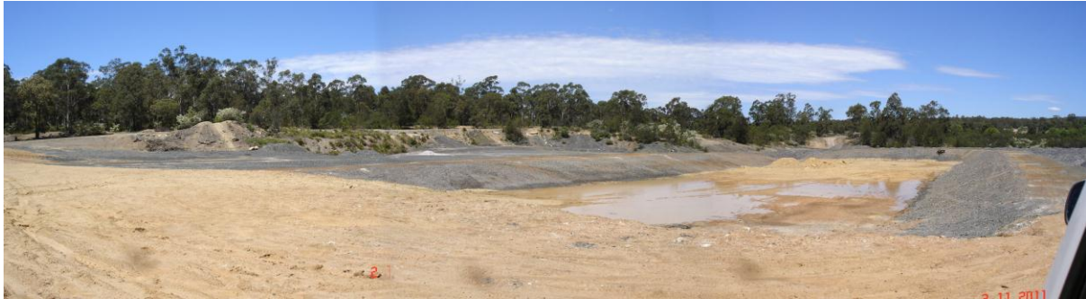
Plate 4.9: Abedare Reject Emplacement Area -nearing completion height for topsoil spreading and revegetation.
