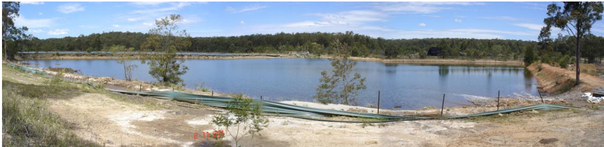
Figure 4.5.2C: Pelton CHPP Water Treatment Ponds
