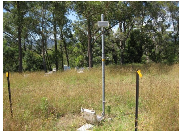
Plate 4.7F: Vibration monitoring station above LW A3
