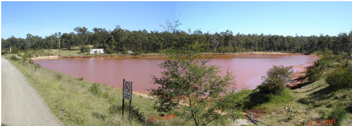
Plate 4.5.2A: Kalingo Dam staging and water storage to assists in the removal of iron and manganese via oxidation
