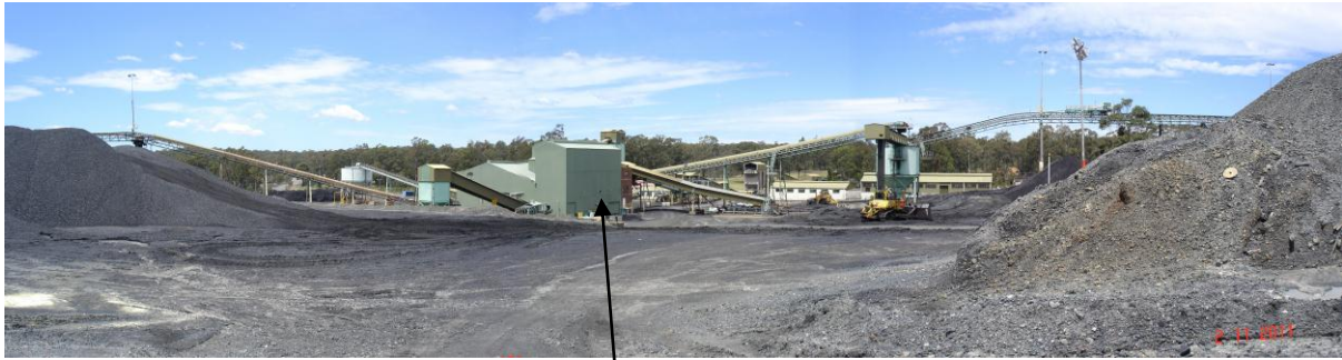
Figure 4.4.3: Pelton CHPP showing new external cladding for noise mitigation.
