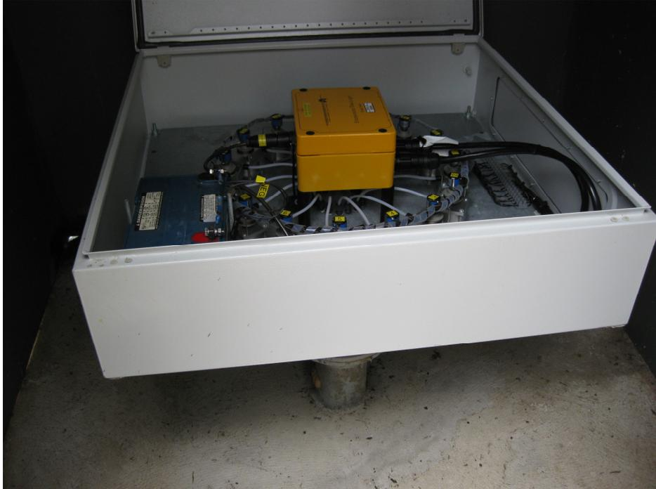
**Photo 8 - Surface Extensometer (AQD 1076) Housing above centre of LWA1**
